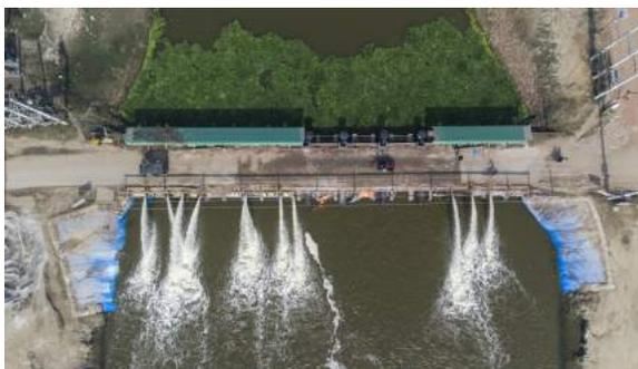
Figure 5: Pumping for removing waterlogging at Bhabadah Regulator
